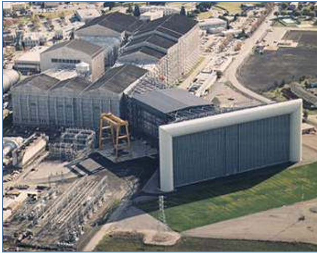
Figure 137: A large wind tunnel facility originally built for circulation through the loop of buildings in background. Entrance cone in foreground was added to also permit once-through operation using the same fans. (NASA)
