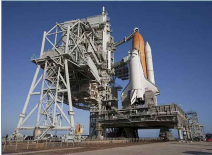
Figure 109: A launch pad with a space shuttle on a mobile launcher platform prior to launch. (NASA)
